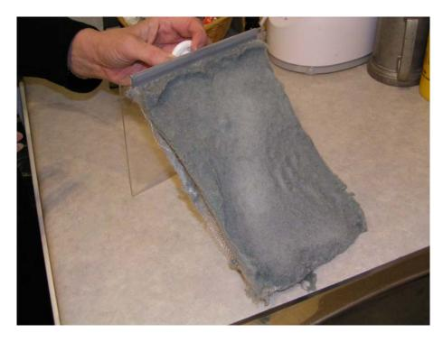
The next picture shows a clean lint-screen, ready for reinstallation in the lint-screen's housing. Nearby, is the pile of newly-removed lint. It obstructs the secondary fan, and it is a fire-hazard.
