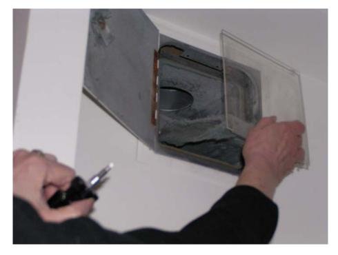
This picture shows the lint-accumulation on the lint-screen's underside. It is about one month's accumulation. Except for creating this mini-manual, cleaning would/should be more frequent.
