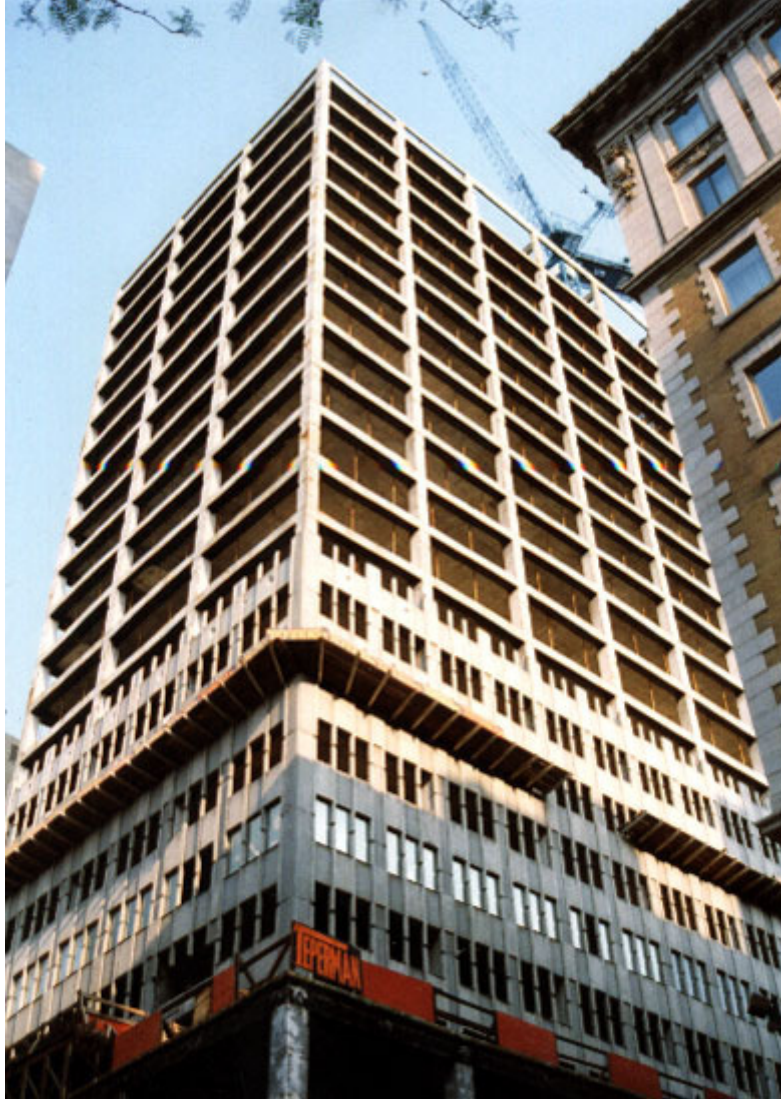
The rear of the building, looking north west.
